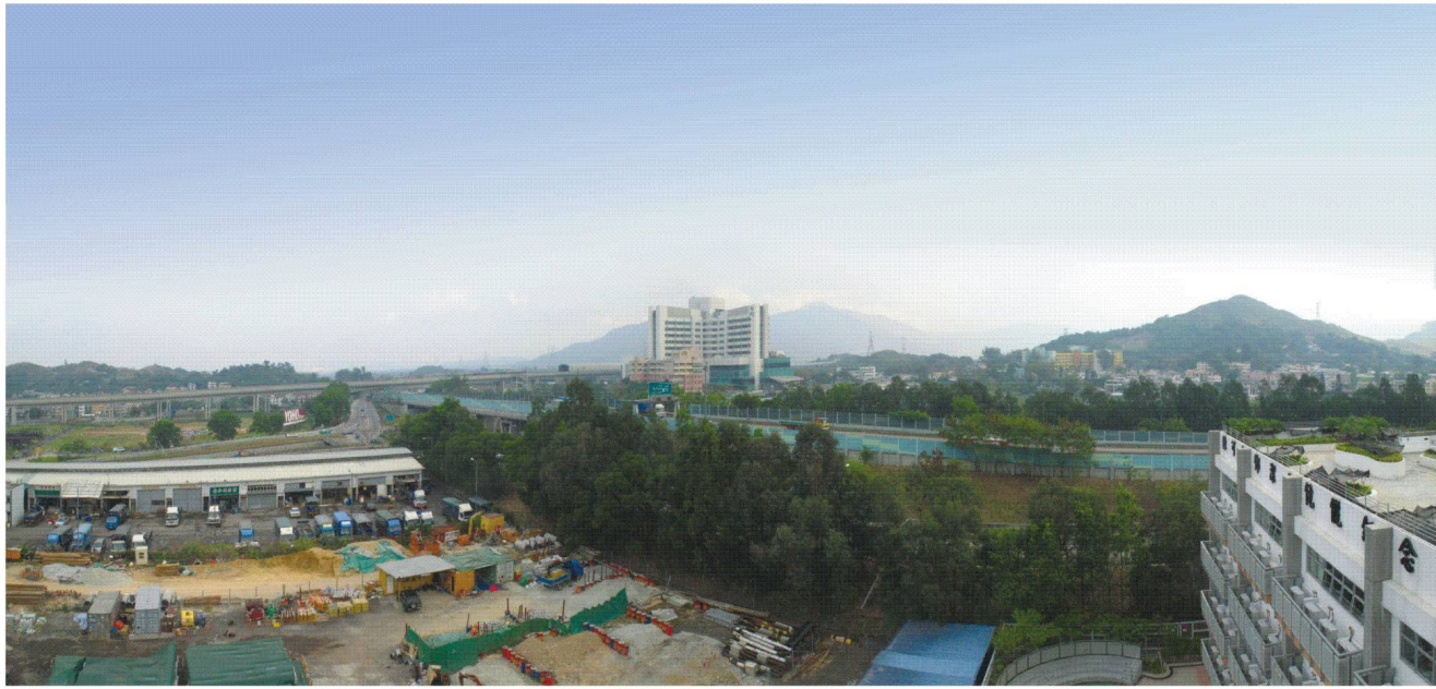
VSR 3 - LOOKING EAST FROM KWONG MING YING LOI SCHOOL: EXISTING CONDITIONS AT THE DEVELOPMENT SITE.
