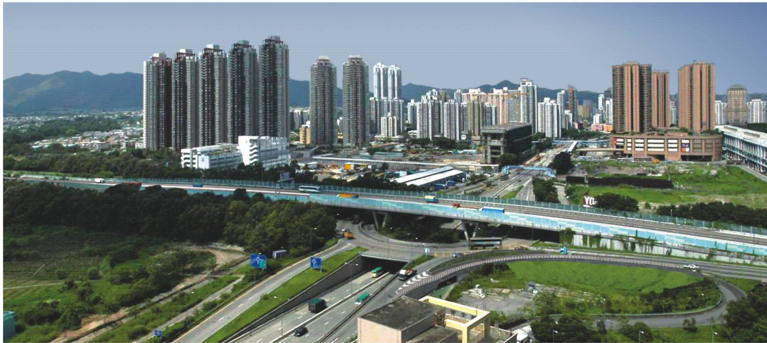
VIEW DISPLAYING THE 3D MODEL OF THE DEVELOPMENT SITE DAY 1 OF OPERATION WITHOUT LANDSCAPE AND VISUAL MITIGATION MEASURES
