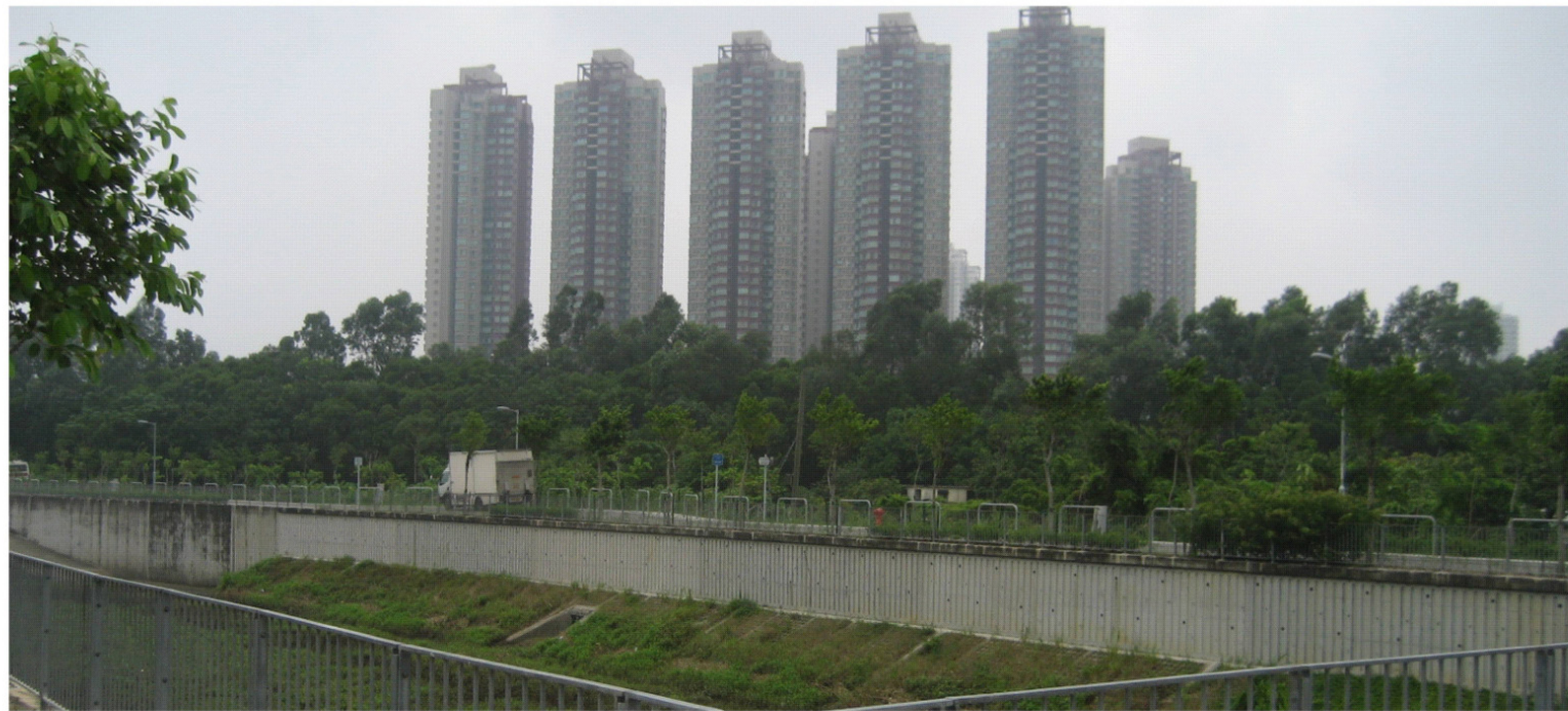
VSR 4- LOOKING SOUTH-WEST FROM YEUNG UK TSUEN: EXISTING CONDITIONS AT THE DEVELOPMENT SITE.
