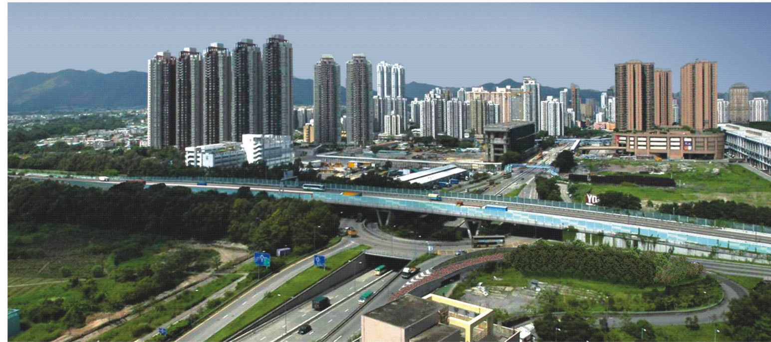
VIEW DISPLAYING THE 3D MODEL OF THE DEVELOPMENT SITE WITH LANDSCAPE AND VISUAL MITIGATION AT YEAR 10.
