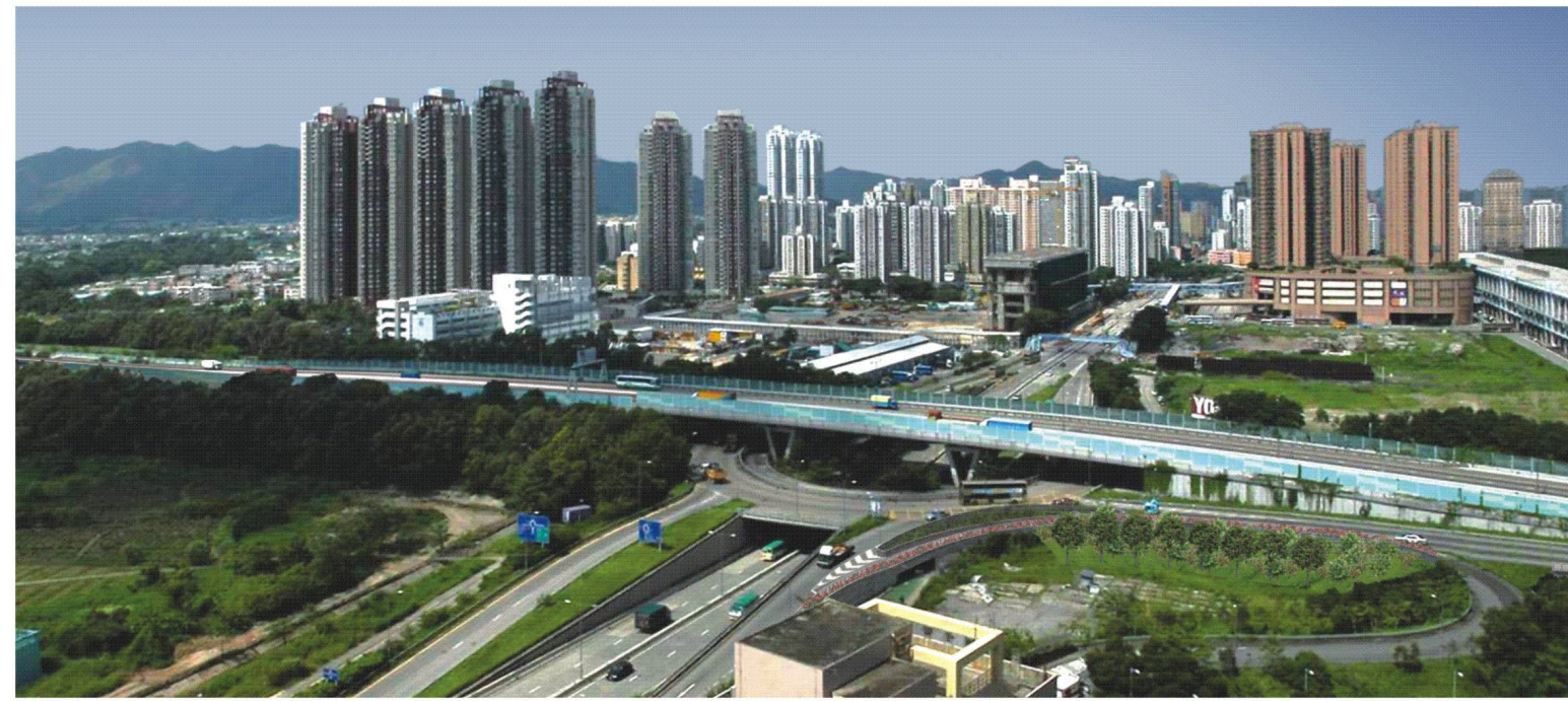
VIEW DISPLAYING THE 3D MODEL OF THE DEVELOPMENT SITE WITH LANDSCAPE AND VISUAL MITIGATION MEASURES AT DAY 1.
