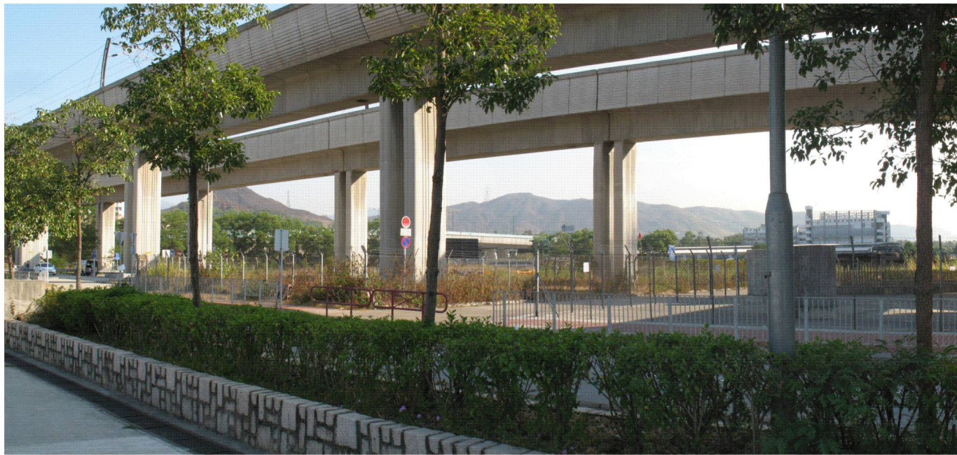
VIEW DISPLAYING THE 3D MODEL OF THE DEVELOPMENT SITE DAY 1 OF OPERATION WITHOUT LANDSCAPE AND VISUAL MITIGATION MEASURES
