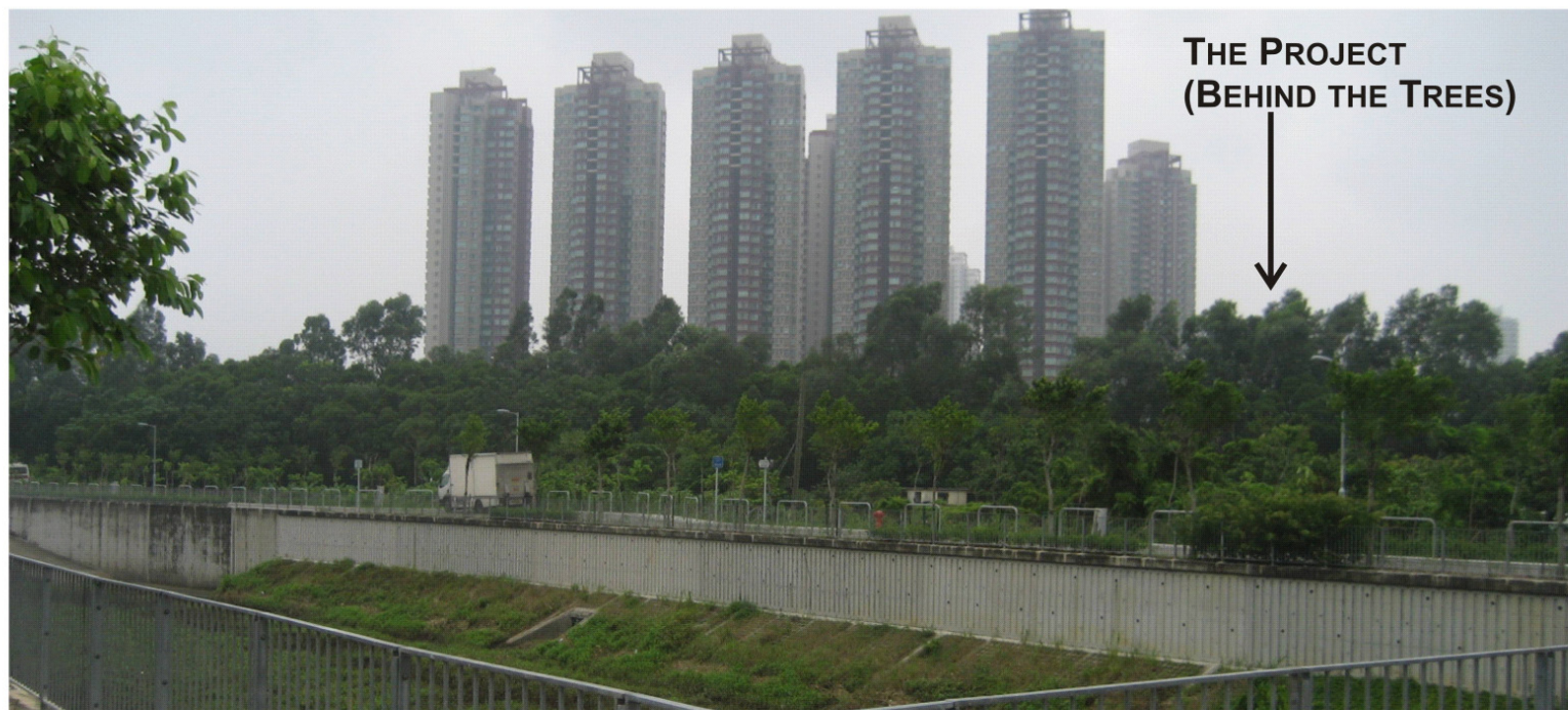
VIEW DISPLAYING THE 3D MODEL OF THE DEVELOPMENT SITE DAY 1 OF OPERATION WITHOUT LANDSCAPE AND VISUAL MITIGATION MEASURES
