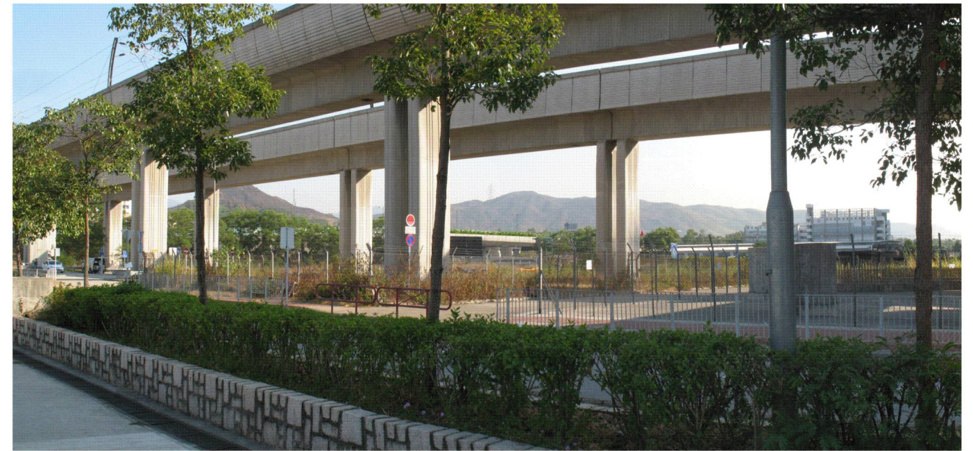
VIEW DISPLAYING THE 3D MODEL OF THE DEVELOPMENT SITE WITH LANDSCAPE AND VISUAL MITIGATION AT YEAR 10.
